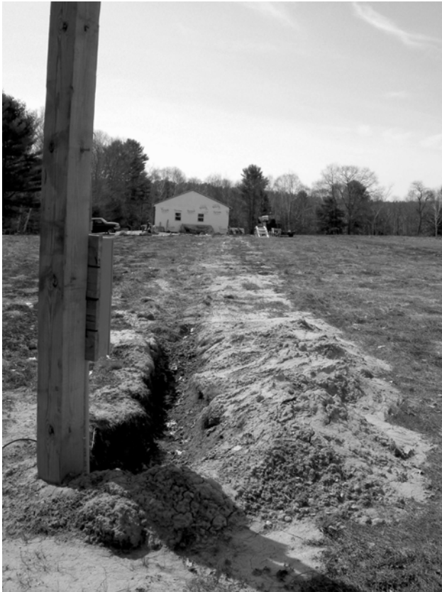
Figure 4. Power pole and powerline trench partially filled in, looking west to the garage on site.
